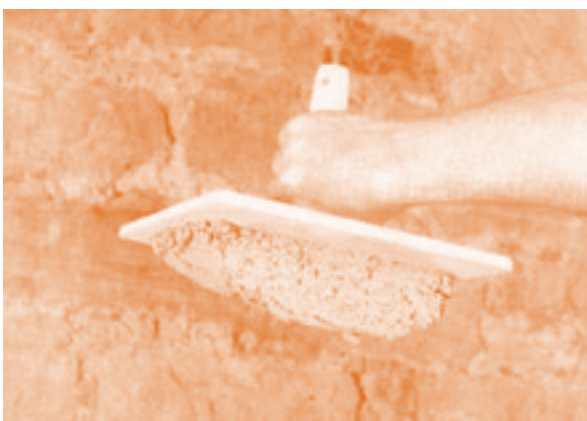
Well made lime mortar will cling to an inverted trowel.
